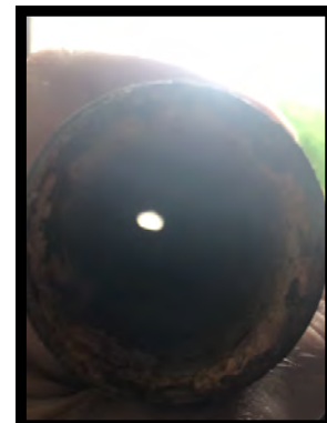
Public Safety water lines were original to the building.
